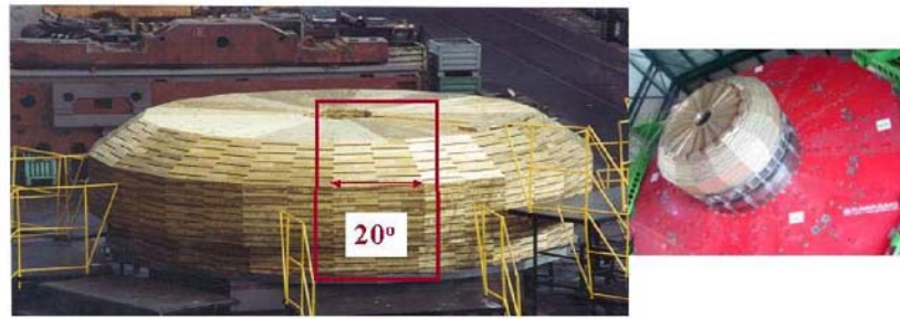
Fig. 5. The end caps are assembled and one of them installed on the end cap iron in surface hall
